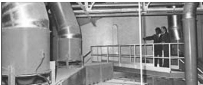
Direct drive duct fans used as part of a process heat and fume exhaust system.
