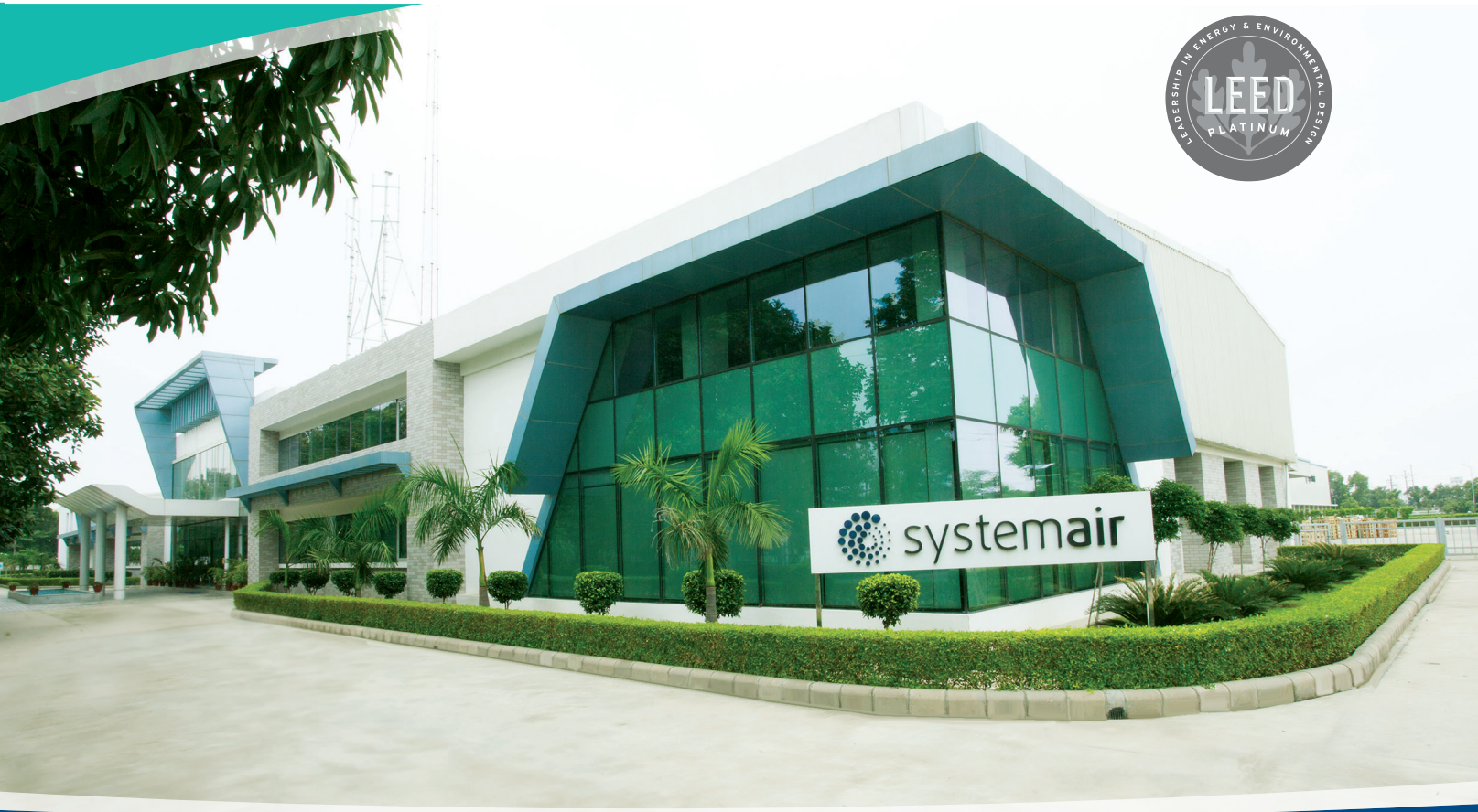
Greater Noida India: LEED Certified Platinum Rated manufacturing facility.
