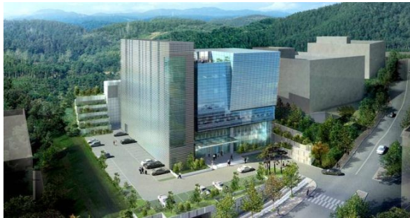
Dongbu hwajae Data Center
