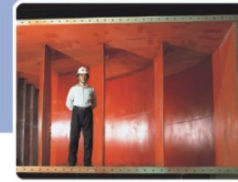
全響室迴風道出口 Exhaust Duct exit of Revererant
