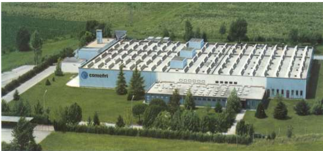
COMEFRI SpA factory at Artegna (UD) – Italy with 68,000 sq.ft. manufacturing and Laboratory floor space for the production of standard and special application industrial fan. Test facilities: laboratory accredited by AMCA.
