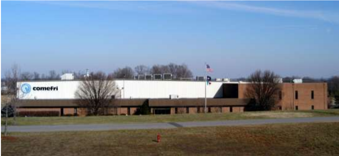
COMEFRI USA: Manufacturing and Warehouse facilities in Hopkinsville, KY. Total facility: 125,000 sq.ft. Producing centrifugal fans for the HVAC industry
