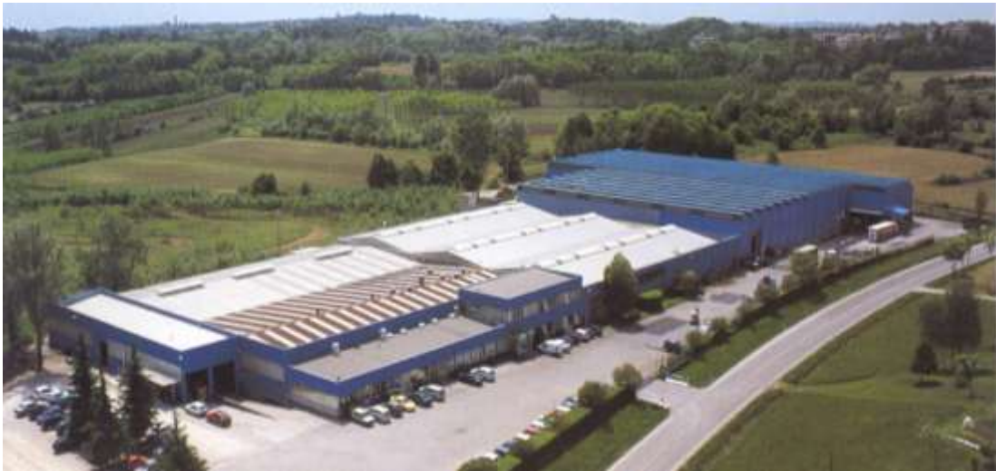
COMEFRI SpA factory at Magnano in Riviera (UD) – Italy with 156,000 sq.ft. Manufacturing floor space, which produces radial fans for HVAC products.
