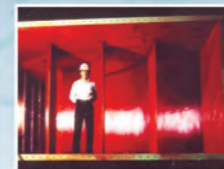
Exhaust Duct exit of Reverberant
