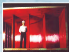
Exhaust Duct exit of Reverberant
