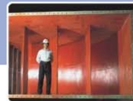
全響室迴風出口 Exhaust Duct exit of Reverberant
