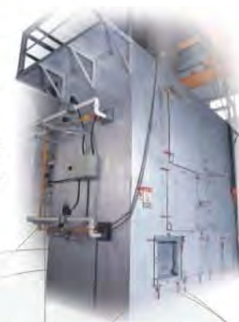
全響室迴風道裝置 Silencer in Exhaust Duct
