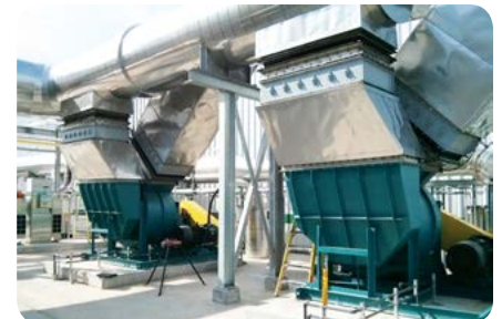
Wastewater Treatment Odor Control
